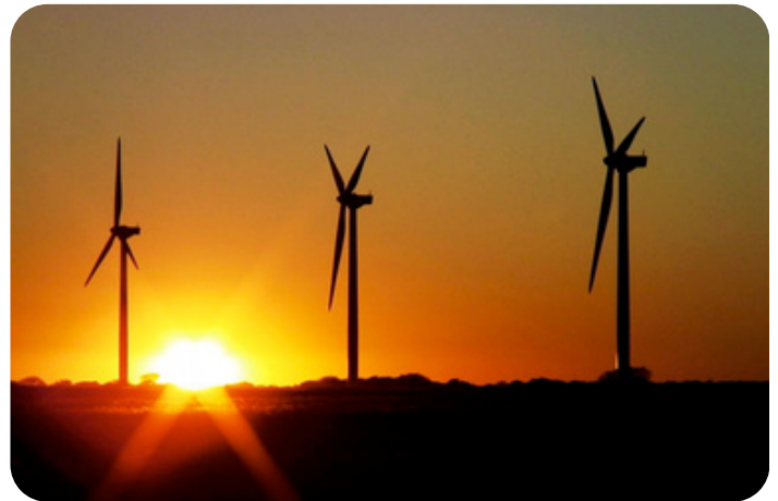
The Gulf Wind Farm in South Texas provides Renewable Wind Energy for Austin Energy's GreenChoice Program.
