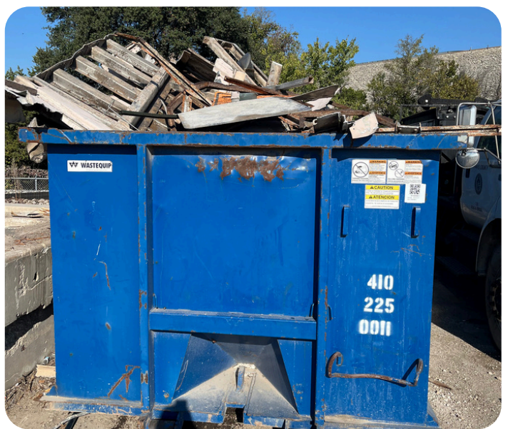
A dumpster filled with metal ready for recycling at the East Service Center.
