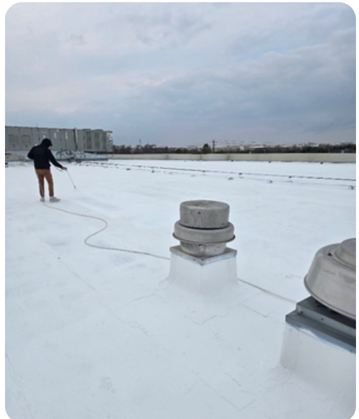
GAF Acrylic Coating is applied to the Pct. 4 Ray Martinez Building (Before and After).
