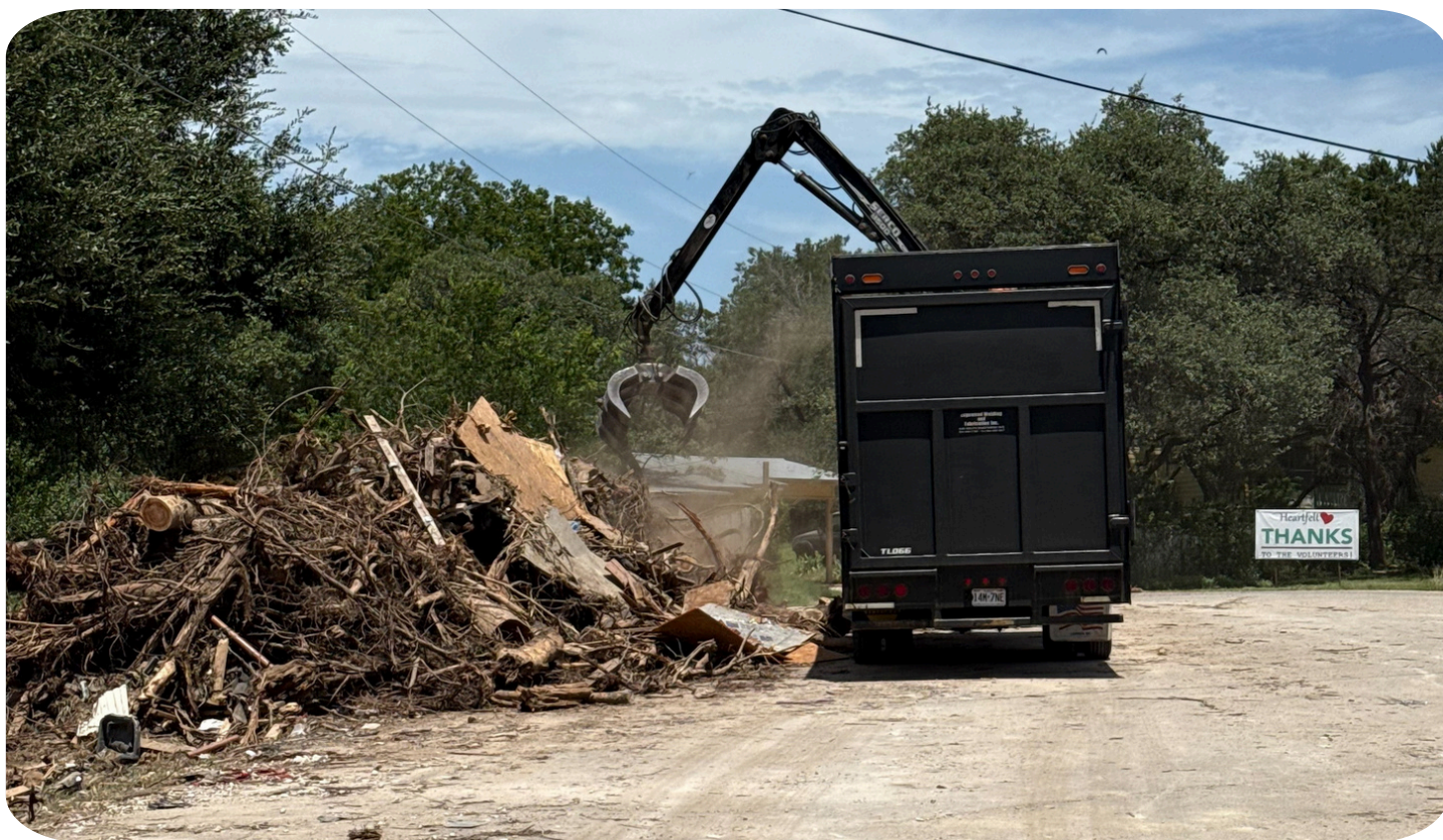
Wood and vegetative debris is collected in NW Travis County near Sandy Creek.
